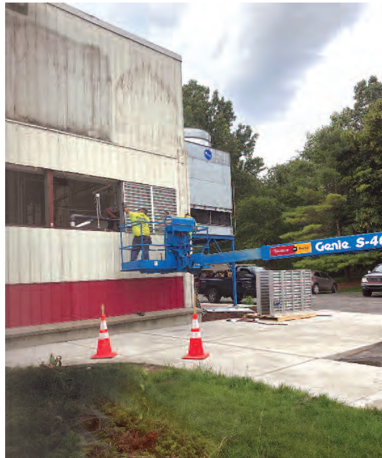
Louver installation in the Mold Room.
