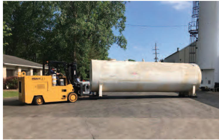
Resin tank removal from the SMC Area.
