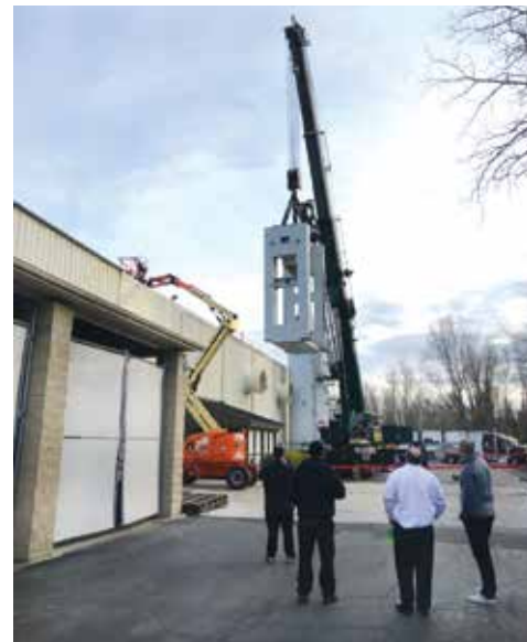
It took a large crane to lift the press and put it in place.
